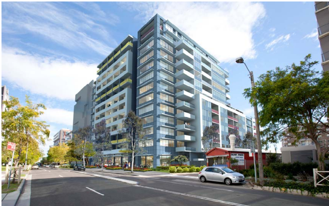
VIEW FROM COWARD STREET COWARD STREET RESIDENTIAL
